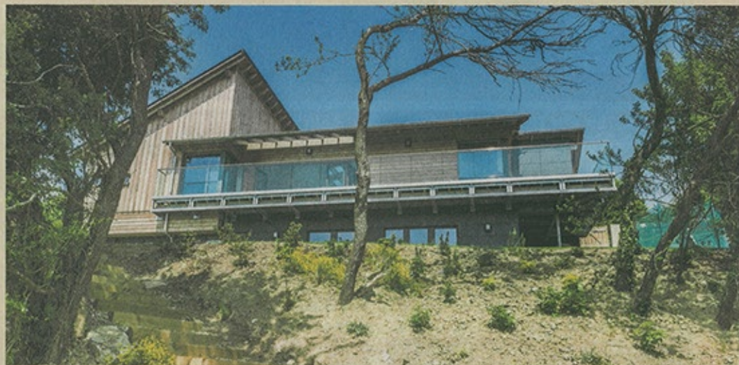
One of the first certified Passive Houses in Cork, sits on the waterfront location in Carrigaline. Designed by Wain Morehead Architects, it was completed in 2010 at a cost of just 3.6pc more — but 1/10th of the heating demand — of a conventional dwelling at the time
