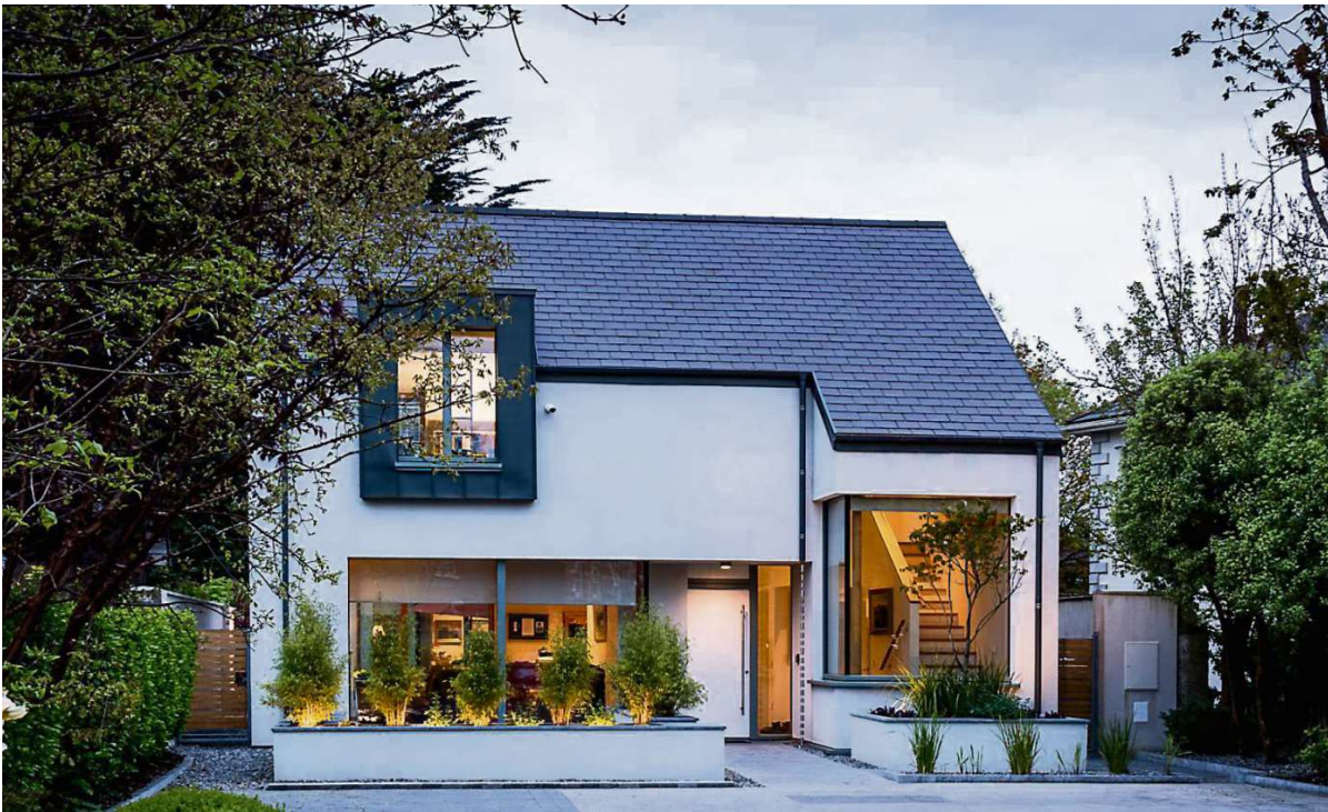
The Douglas Road home which is the first house in Ireland to achieve Home Performance Index gold certification from the Irish Green Building Council.
